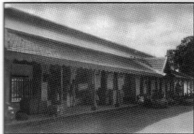
Dilawar Gadh Railway Station Jetpur
